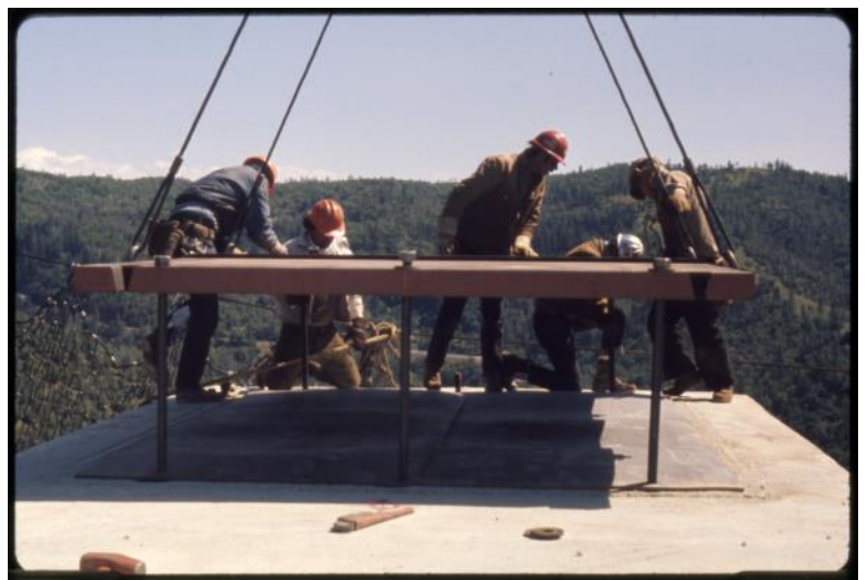
Foresthill Bridge Construction, c. 1972.
