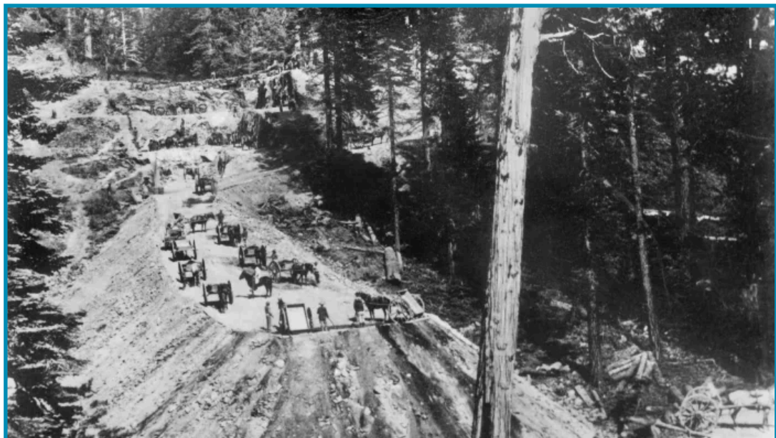
Chinese workers building a cut and a bank at Sailor's Spur in the Sierra foothills for the Central Pacific Railroad in California, 1866.
